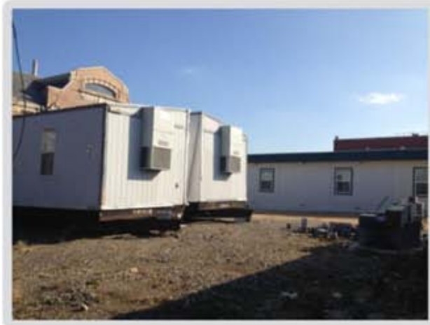
6 TEMPORARY OFFICE TRAILERS - WEST ELEVATION
