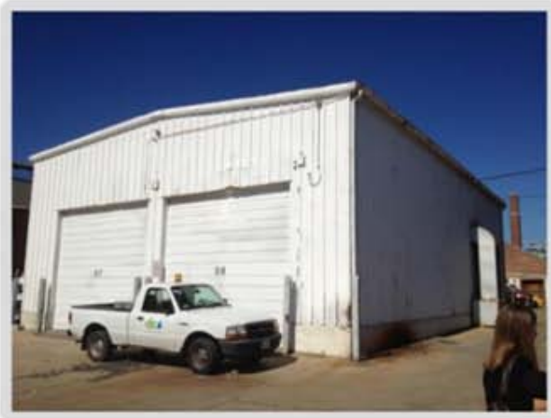
4 PAINT SHOP - SOUTH ELEVATION
